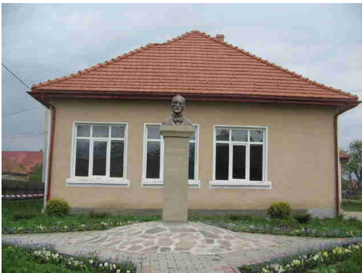
Elementary school in Szentatolna.
